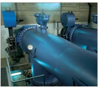
Vertical cylinder downward, clockwise closing VAG EKN® 48" Butterfly Valve with HYsec Hydraulic Brake-and-Lift Cylinder, installed in the Eibenstock dam in Germany.
