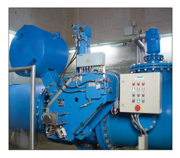
Vertical cylinder, anti clockwise closing VAG EKN® 48" Butterfly Valve with brake and lift cylinder, installed in the Leibis-Lichte dam in Germany.
