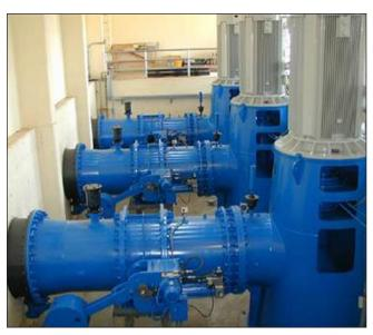
VAG EKN® 54" Butterfly Valve with HYsec for water supply at a plant in Poland.
