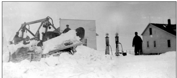
All that snow! "Metzgerville" signage not yet painted on the building.
