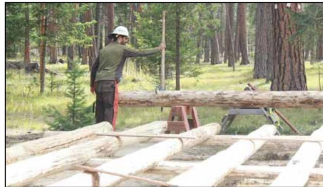
**Using a cant hook to turn the logs. In the foreground the floor joists are laid.**
