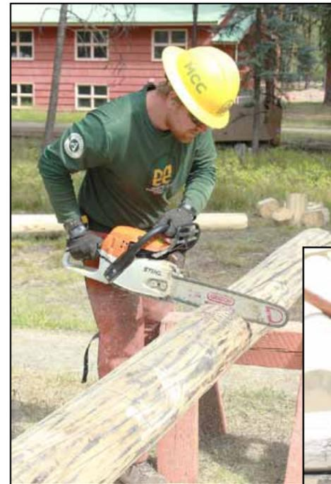
**MCC crew member sawing a rough V-notch (above) and chiseling a rough notch (right). The crew was first taught using only hand tools. They switched to chainsaws to speed up the process.**
