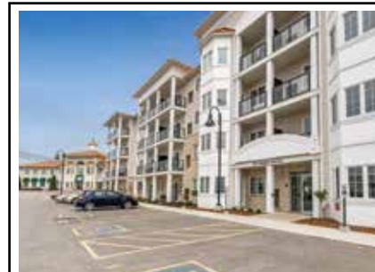
105-80 Shipway Ave, Newcastle
