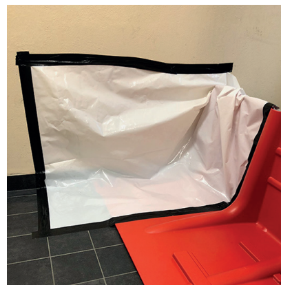
Using a piece of liner for sealing
