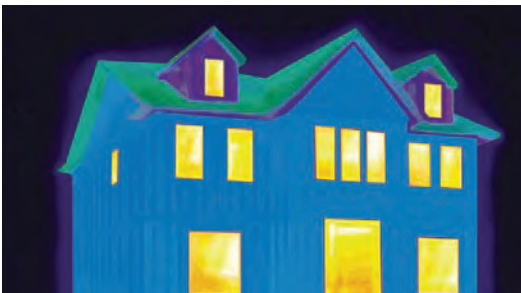
Thermal imaging shows the notable difference in heat loss between an exterior wall that relies on stud walls with cavity insulation (top) and a wall that uses continuous insulation (bottom).
