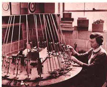
One of a battery of fletching tables where both stock and custom arrow fletchings are assembled on special, Hoyt designed, Tri-Heli-Fletchers.
