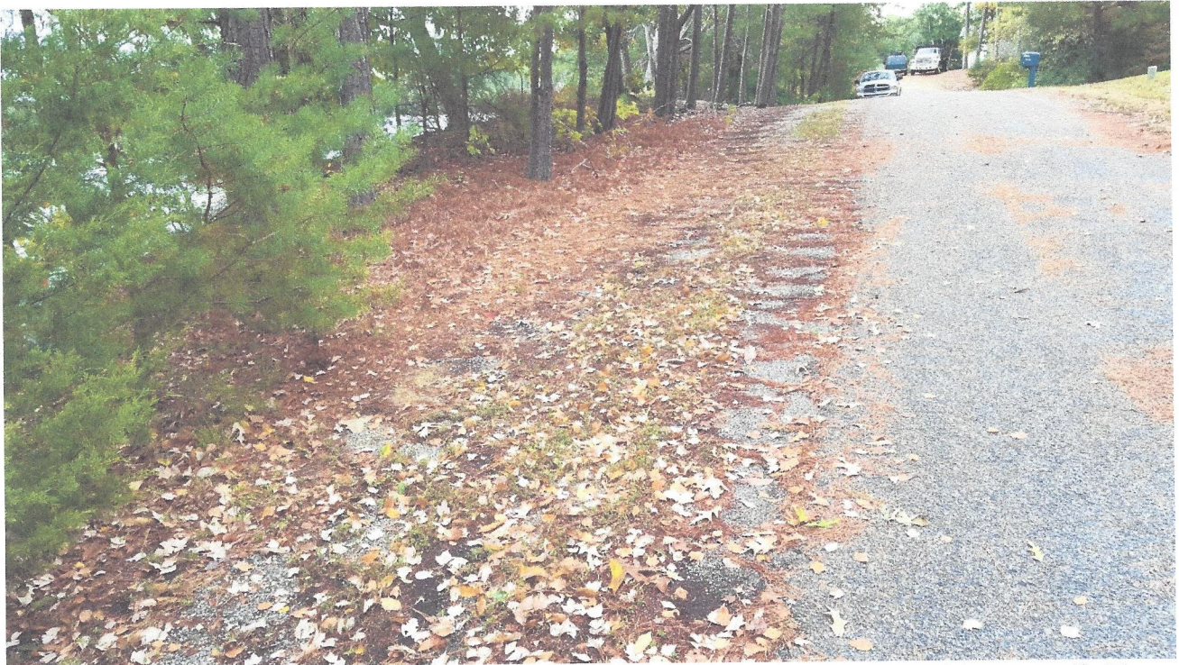
Photo 1. Development Road and Top of Evaluated Properties Shoreline Bank. Note runoff rills.
