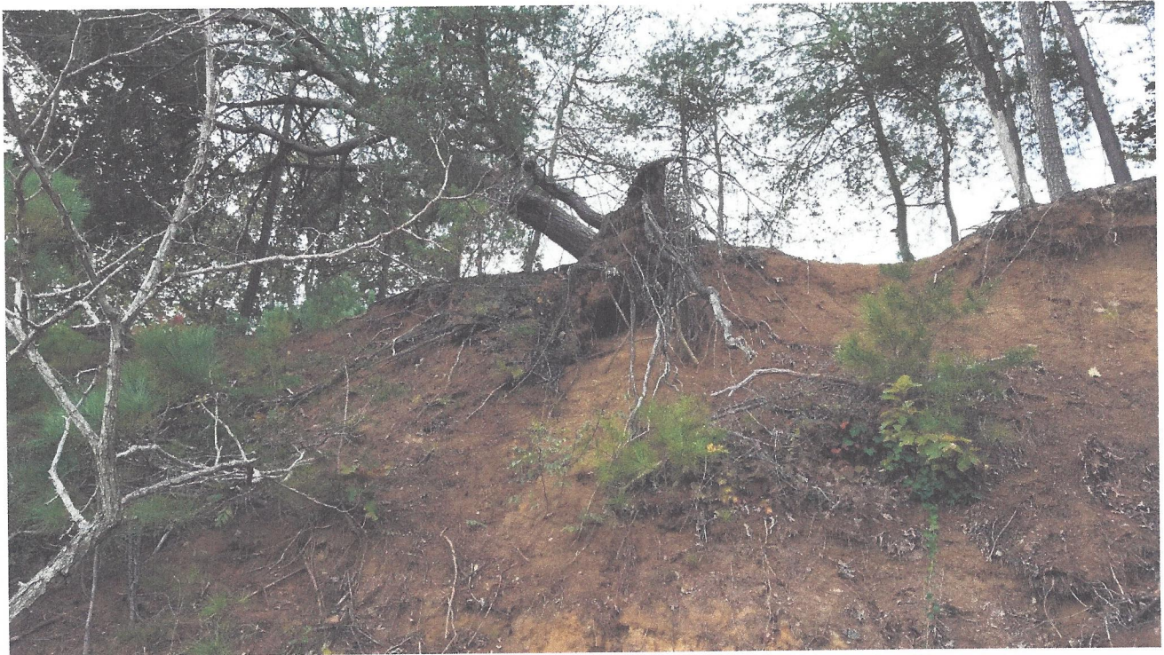
Photo 2. Lot 3a & 4a Upper Slope erosion and loss of Protective Veneer and Vegetation.
