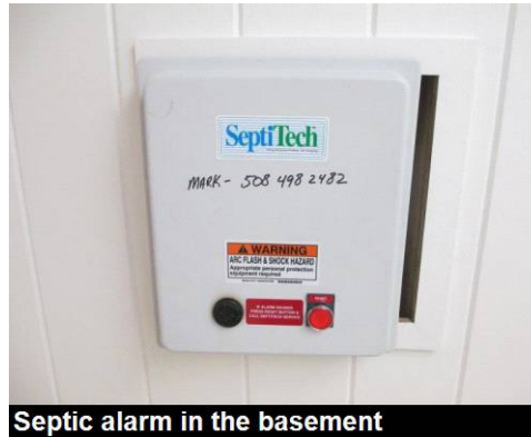
Septic alarm in the basement
