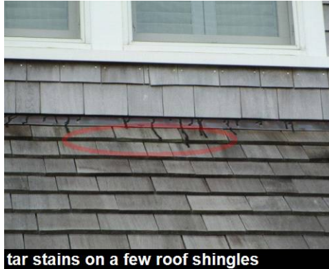
tar stains on a few roof shingles
