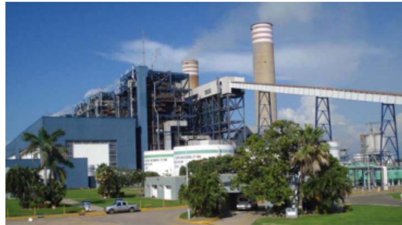
Comisión Federal de Electricidad's Petacalco Power Station in Mexico
