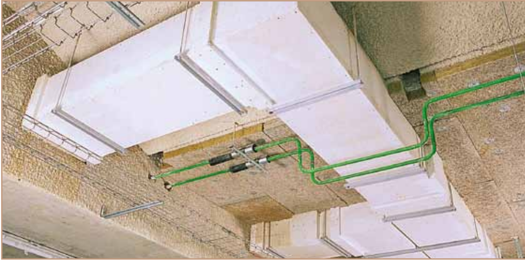
Example of application: ventilation and smoke extraction ducting.
