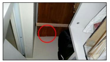
**37. Condition:** • Holes are visible in the ceiling and wall. Patch and repair as needed **Location**: Basement Bedroom closet
