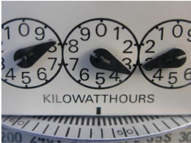
This type of electric meter works on the eddy current electrical principle. The silver disk you see protruding through the slot with black bars is actually made of aluminum. This disk is the visible part of an electric motor inside the meter known as the rotor. In electrical motors the rotor is made of a magnetic steel alloy which is required for the motor to rotate. Yet in older electric meters the rotor is not magnetic. So how can it work at all?
