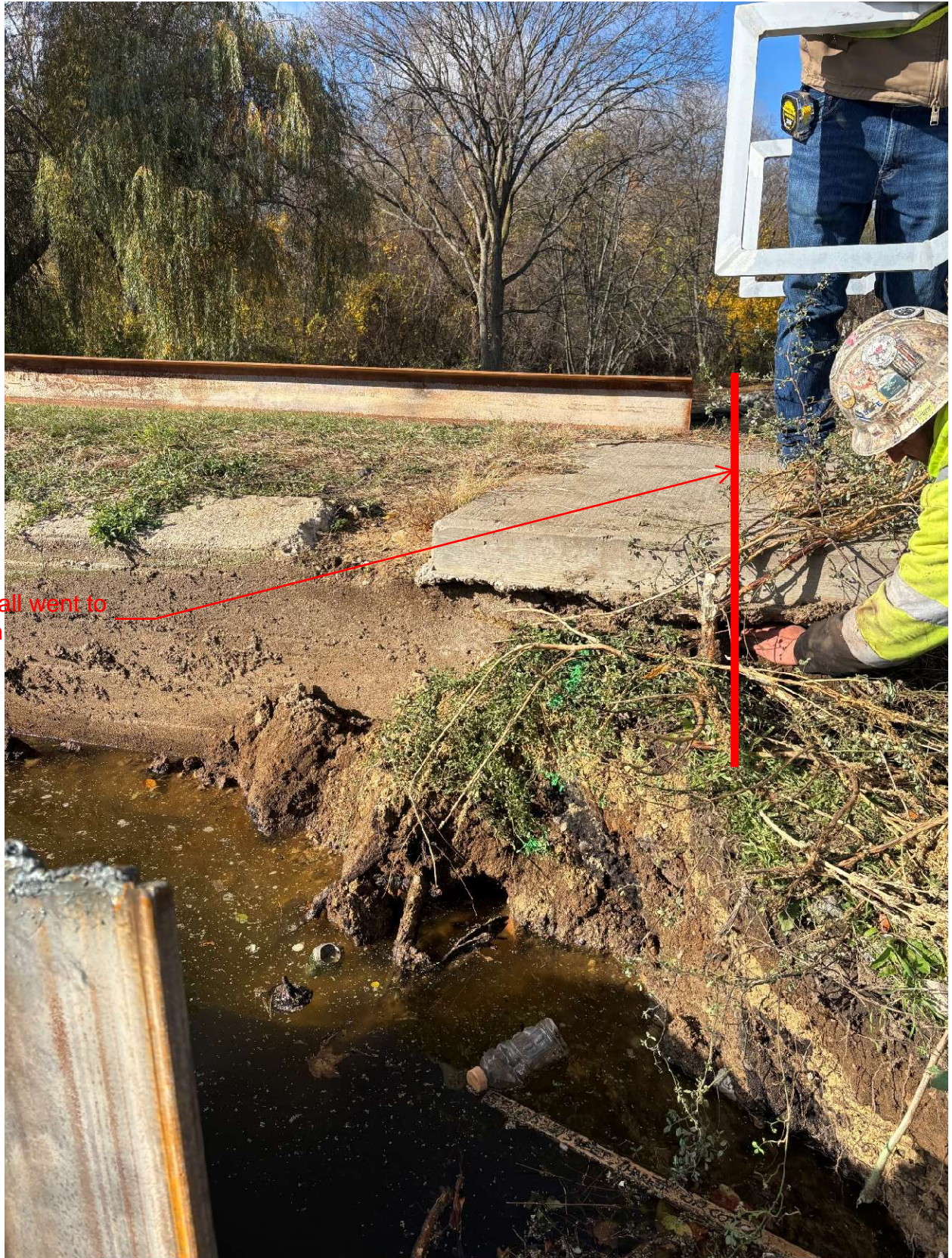
Figure 1: Existing concrete wall fail underneath the existing stoop.
