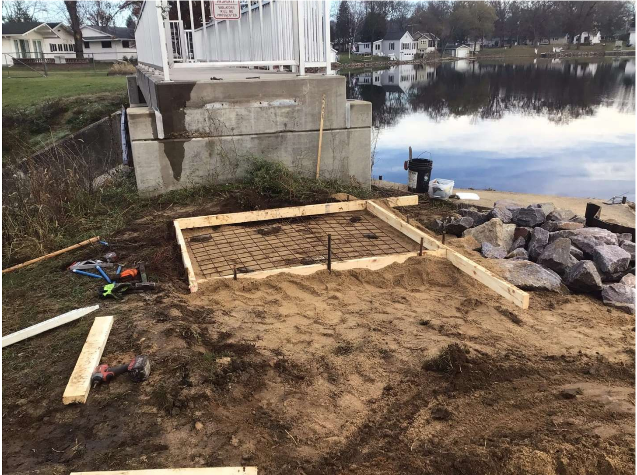
Figure 2: Concrete stoop during construction.
